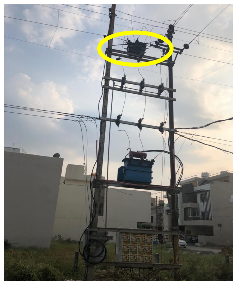
Figure 18. Metering on Repaired 100 kVA DT
