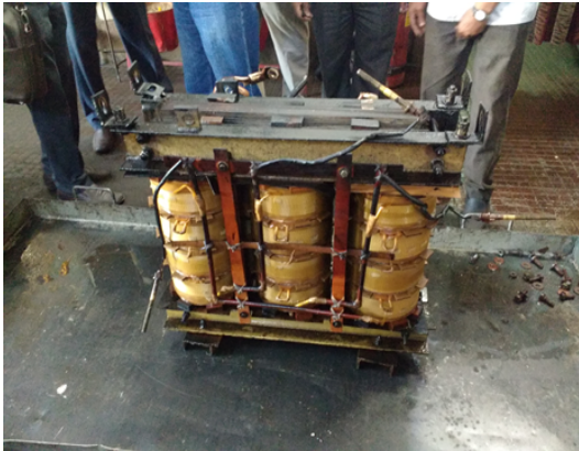
Figure 1. Acquired failed DT
